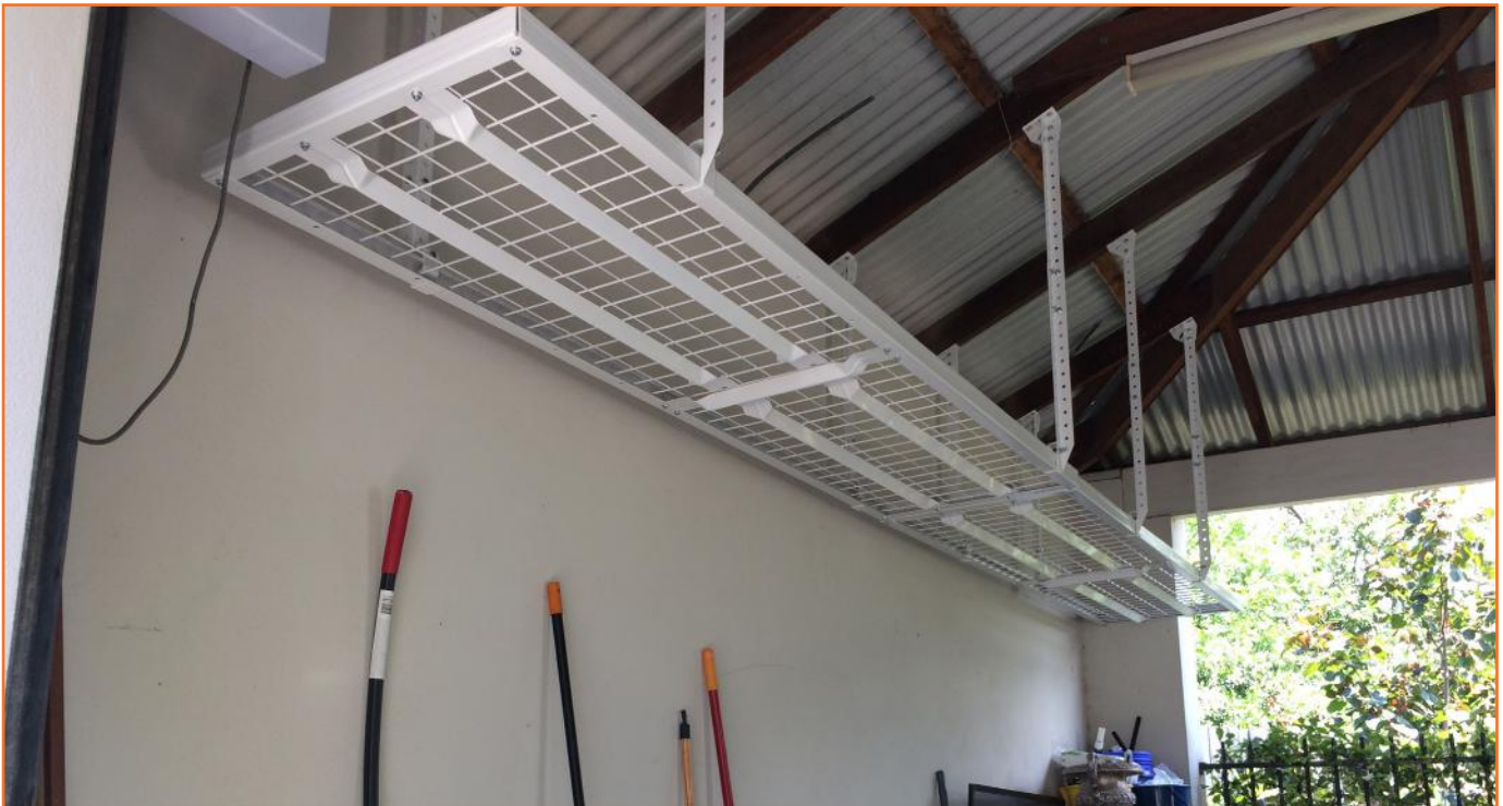
Two SuperPro units suspended from sloped ceiling beams
